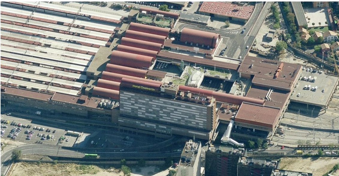
Figure 2: Aerial view of HUSA Chamartín Hotel and Railway Station
